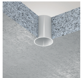
Fig. 5: Permanent formwork for rigid floor
